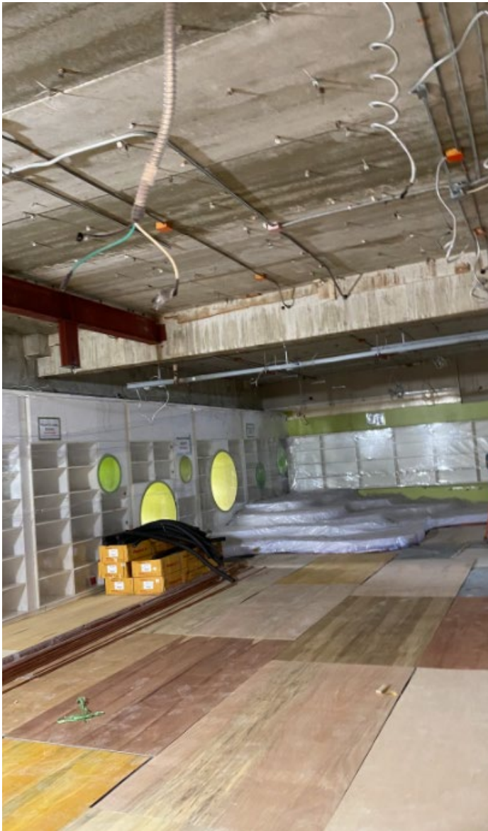
The HUB ceiling was removed and replaced over the summer.
